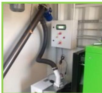
A correctly sized biomass boiler installation should heat the commercial or domestic requirements with a design temperature below freezing, however for at least 80% of our heating periods, the ambient temperature is far higher. By cascading several boilers together, only the energy required at the relevant time is provided.
